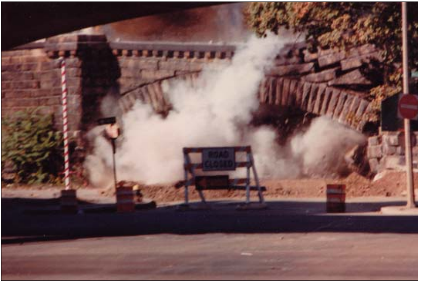
Implosion of Forest Hills Viaduct, November 1983. Photograph by Richard Heath
