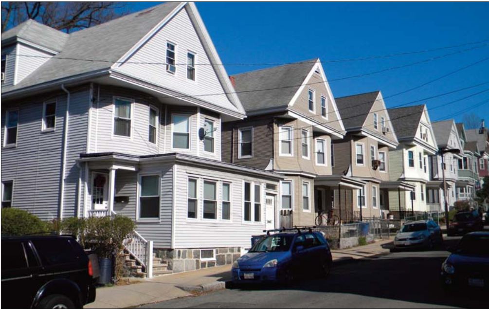
Weld Hill Street homes, built 1894 - 1895. Photograph by Richard Heath
