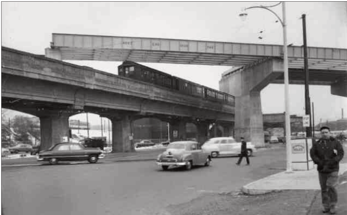
Construction of the Casey Overpass at Forest Hills in 1953. Jamaica Plain Historical Society Photo Gallery. Anthony Sammarco photograph.
