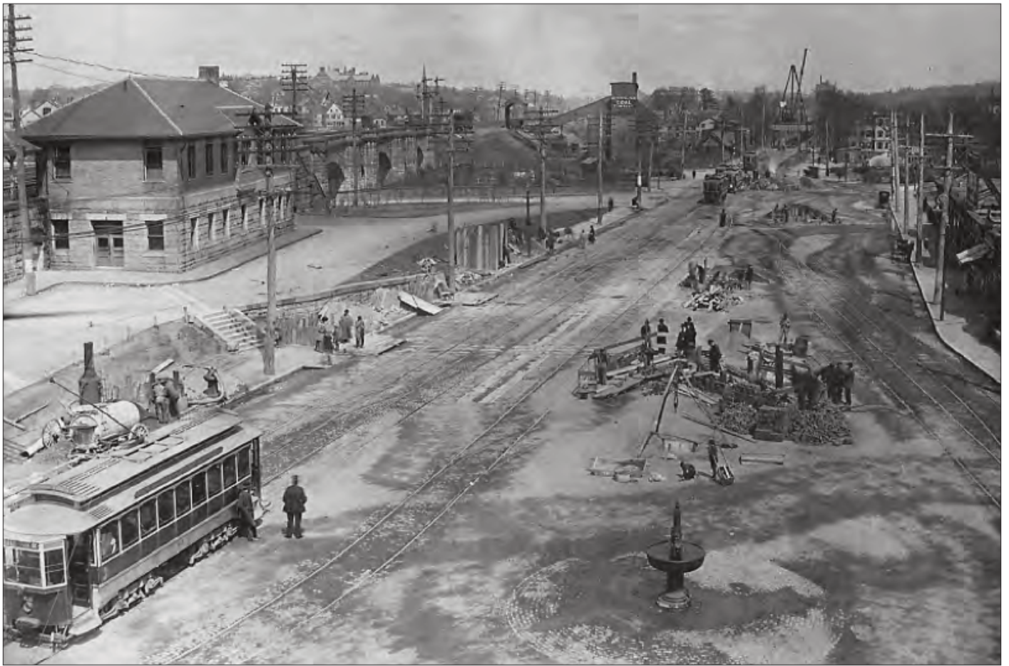
Construction begins on Forest Hills Terminal 1908. Photograph from Rollsign, September - October, 1984.
