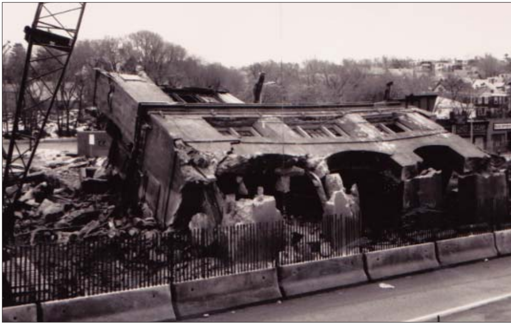
Demolition of Forest Hills terminal February 20, 1988. Photograph by Richard Heath
