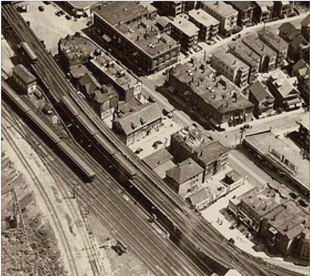
1929 aerial photo. Detail showing the Morton block oval with Tollgate Inn and Forest Hills Hotel. Boston Public Library Print Department
