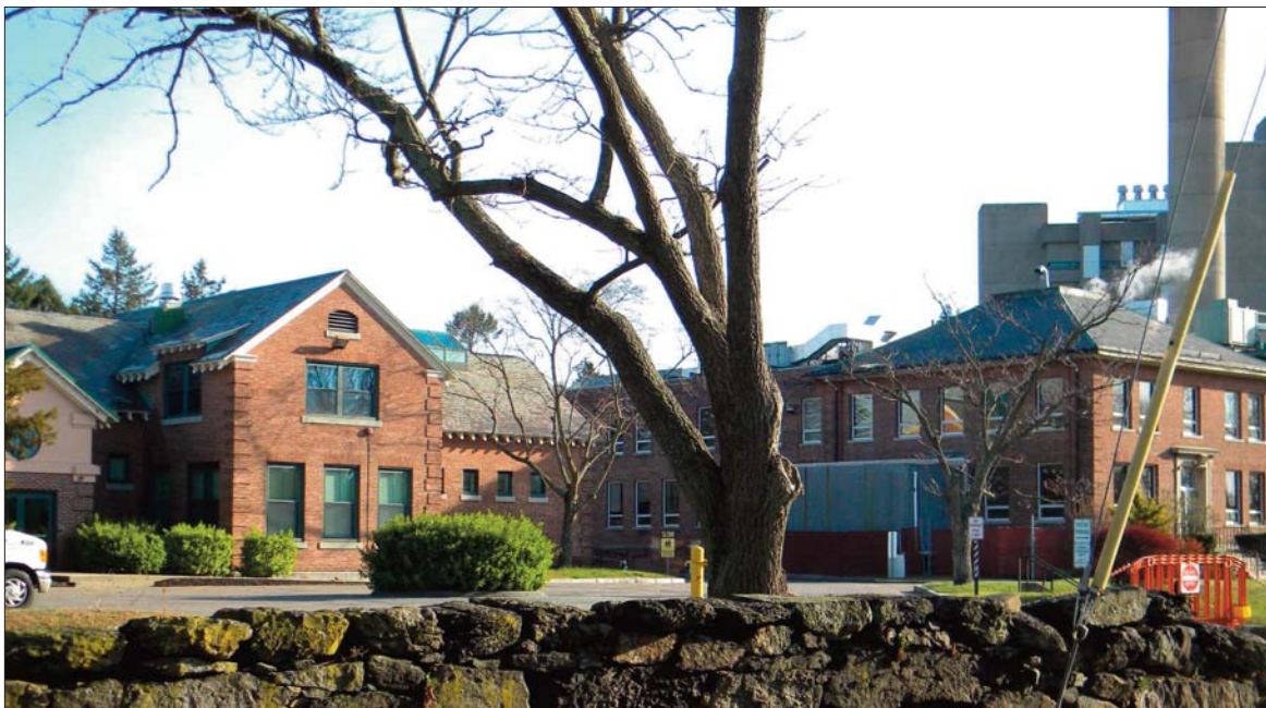
Remaining buildings of the Bussey Institute with original boundary wall on South Street. Buildings built in 1905, including the stable on the left. Photograph by Richard Heath
