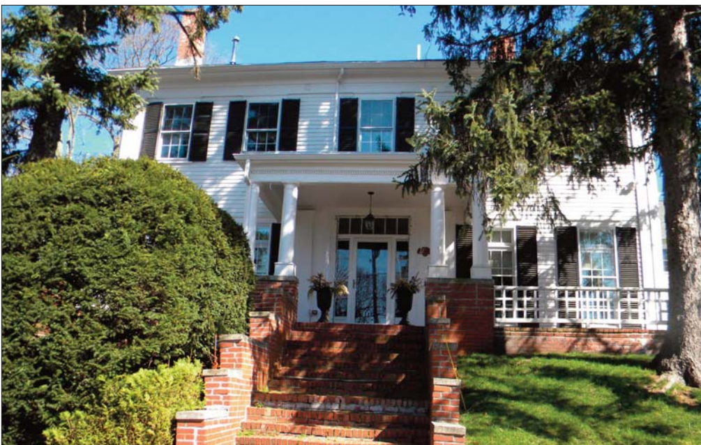
40 Orchardhill Road. Built about 1849. Photograph by Richard Heath
